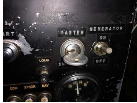
Master Switch – shown in 'on' position Rotate 90 degrees left to 'off' Key will be vertical when 'off'
